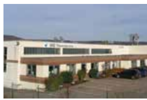
AKG Thermotechnik GmbH & Co. KG Uslar, Germany
