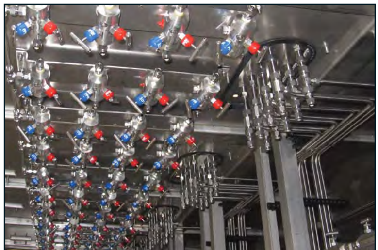
Installation Picture using our Standard Range of Ball and Needle Valves
