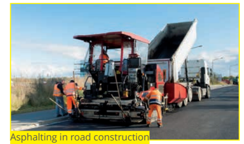
Asphalting in road construction
