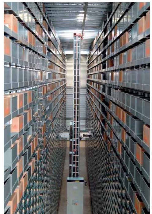
Fully automated high rack warehouse
