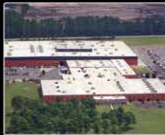
CONWAY, SC Steel Foundry and Manufacturing Plant
