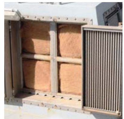
▲ Dust-loaded TI-APM blankets
