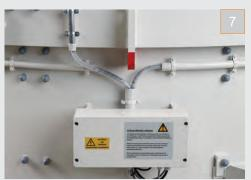
7 | Electrical components are completely pre-wired to an electrical junction box.
