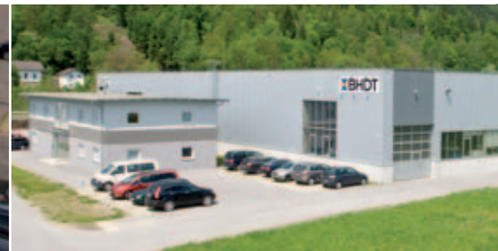
BHDH Pump Production and Welding Center, Hoenigsberg
